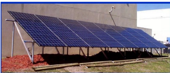
Figure 14: Ground mounted solar modules
