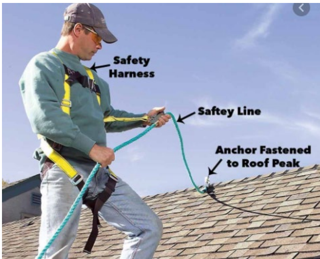
Figure 25: Safety working on roof (pinterest)
