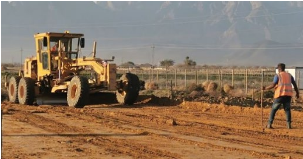
Figure 36: Site preparation ( https://amandlaconstruction.co.za/ )
