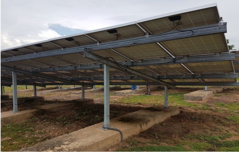
Figure 37: Ground Mount installation, Foundation example
