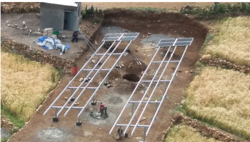
Figure 39: Foundation work, SEF
