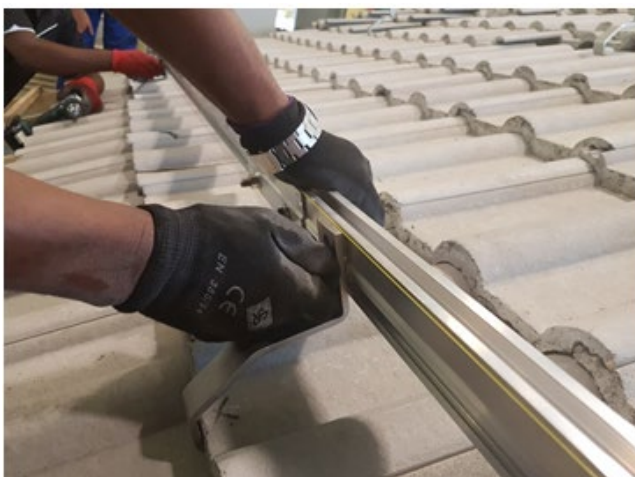
Figure 82: Mount the rails
