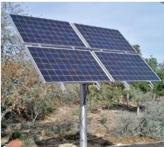
Figure 70: Pole Mounted System ( https://cuttingedgepower.com/ )
