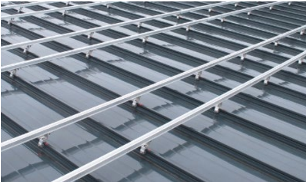
Figure 63: Rails mounted onto seamed roof clips ( https://rooftech.de/ )
