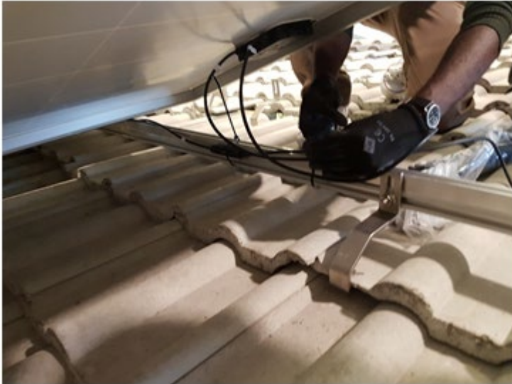
Figure 83: Tying up the cables
