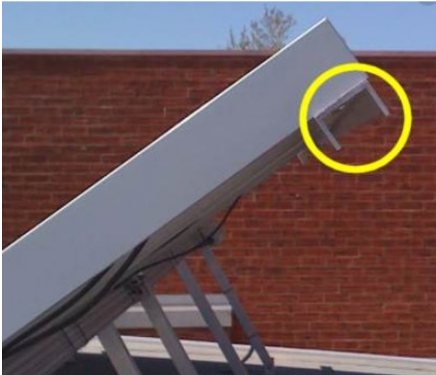
Figure 73: Solar Panel bolted to frame
