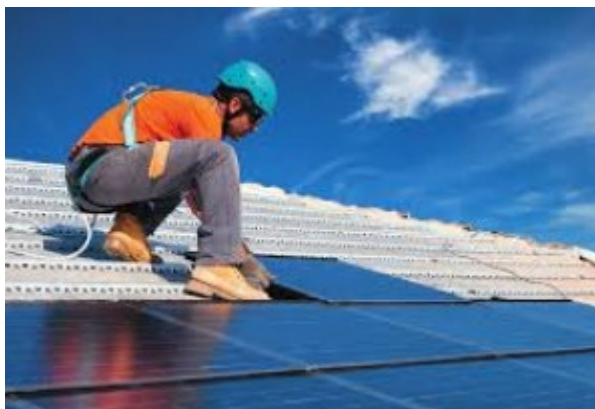
Figure 7: Working at heights (internet)
