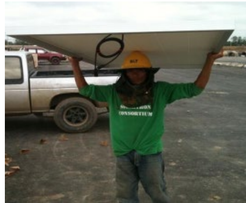
Figure 37: Wrong way to carry a module
