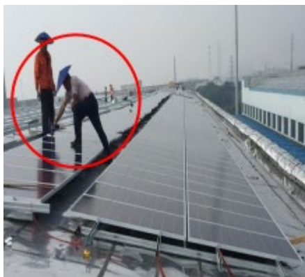
Figure 3: Do not walk on modules
